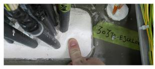
After sealant has cured, use a non-sharp object or your thumb and press into the sealant to detect if at any point the object/thumb penetrates the sealant which would indicate the thickness of sealant is not achieved. Alternatively, a knife can be used to carefully cut away a small piece of the sealant (i.e.20x20mm or 0,8") and then verify the min thickness of 15mm (0,6"). Reseal with Marine Flex Sealant.
