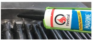
Finaly, re-seal the hole where the nozzel was inserted with Marine Flex Sealant.
