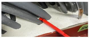
Inspect that the cables are separated between each other and from cables to sleeve with a distance of min 5 mm (0,2").
