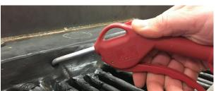
Insert an air hose with a nozzle (with appropriate O/D) through one side of the sleeves silicone layer and apply air pressure of maximum 0,1 bar (1,45 PSI).
